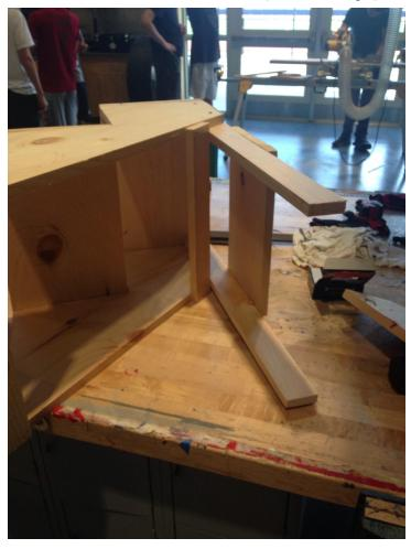
Our last step was to make legs for the stairs so they could stand by themselves and then add extra support boards on the bottom to help reduce sway and provide extra support for the overall structure.
